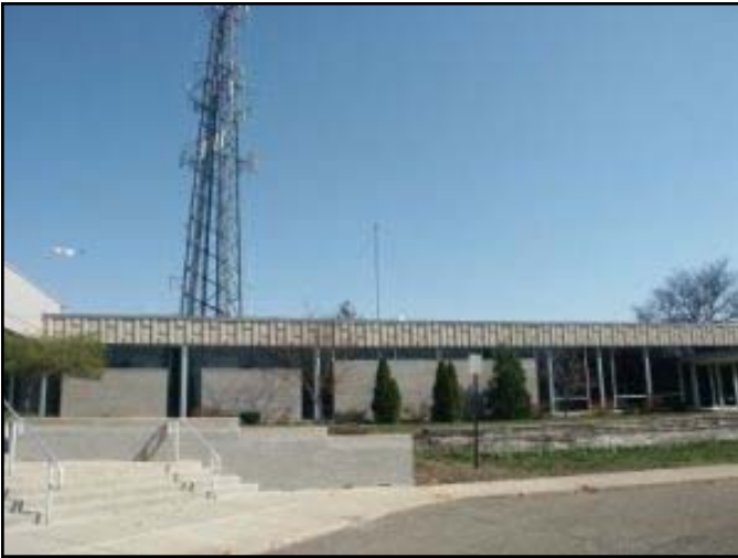
Center support for the 80 Meter dipole in the shadow of the LPD tower. The dipole was used for CW.
